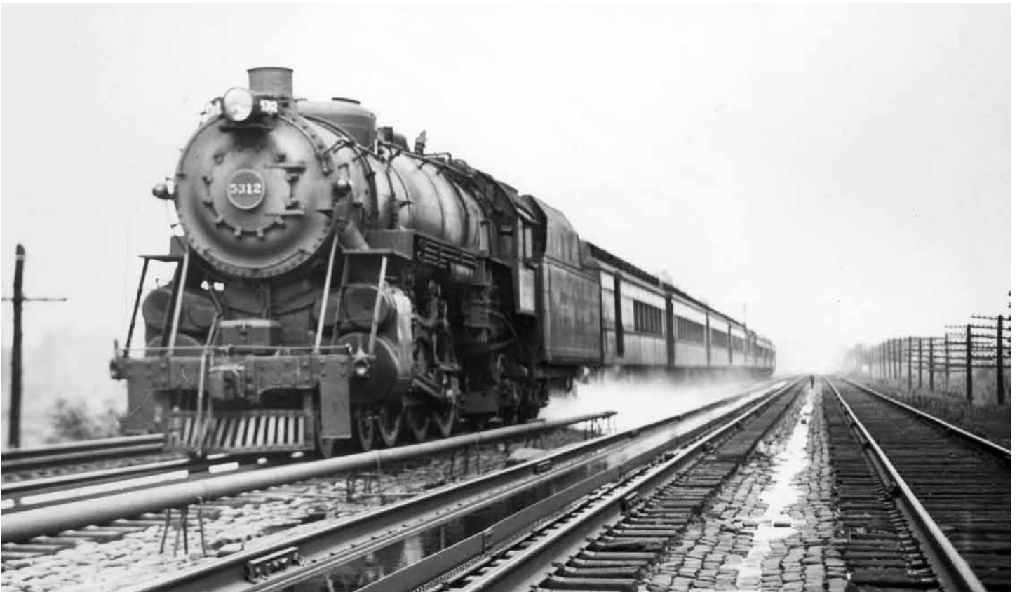
The Columbian is westbound at Green Brook (Middlesex, New Jersey) on the Central of New Jersey. Penstocks were provided on the two outer tracks for freights. The pipe between the tracks, held off the cold ground by metal supports, is for steam heating in winter. The Belgian block used for drainage is apparent between the two eastbound tracks.
