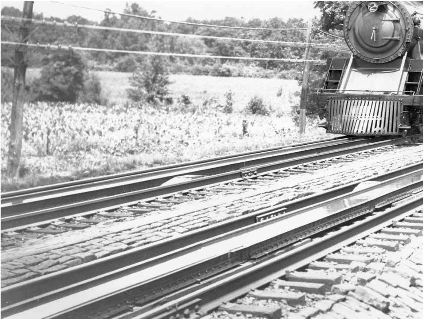
The track pans sat in a one-inch pocket milled out of the ties. Riveted to the side was a bracket that was spiked to the ties, allowing for expansion and contraction. Belgian block paving provided protection to the roadbed and better drainage of the spray kicked up by the water scoop. The block had once been used for the driveway of the freight shed in Pittsburgh.
