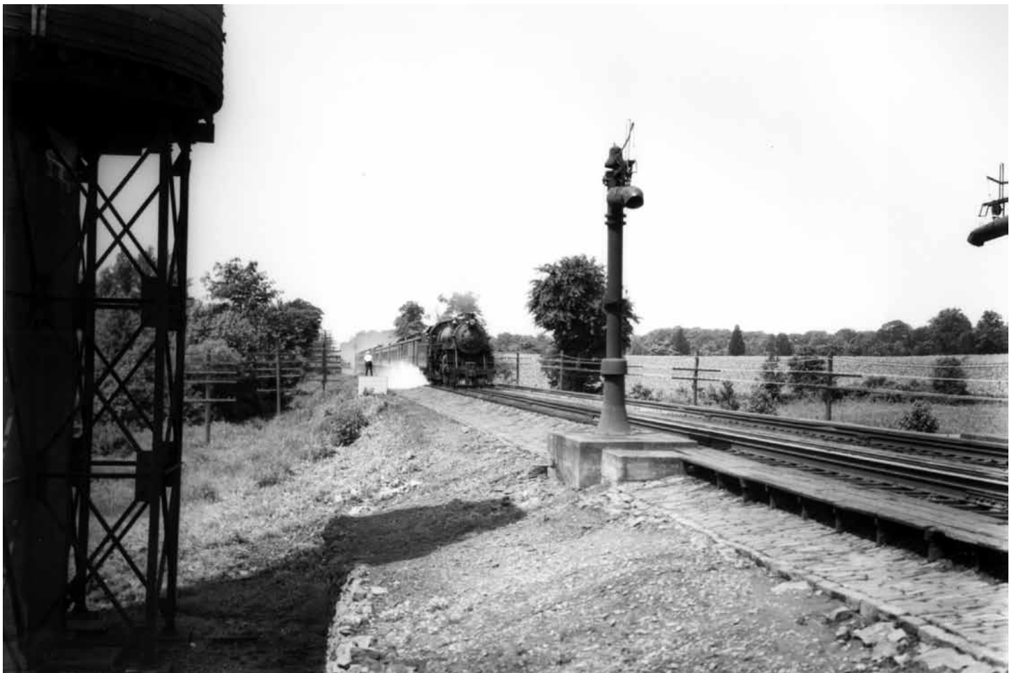
Penstocks were provided at both water stations—Swan Creek and Stanton—for freights, which did not scoop. They were also a backup for passenger engines in the event of a track pan or scoop malfunction. The storage tank at Swan Creek is in the left foreground. The train is eastbound.
