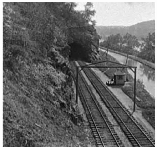
West portal of B&O Railroad tunnel at Point of Rocks, Maryland, circa 1892.
