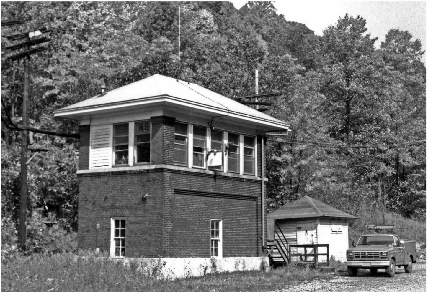
West End (WS) Tower just west of Kingwood Tunnel, West End, West Virginia. (Gary Schlerf photograph, B&O Railroad Historical Society Archives)
