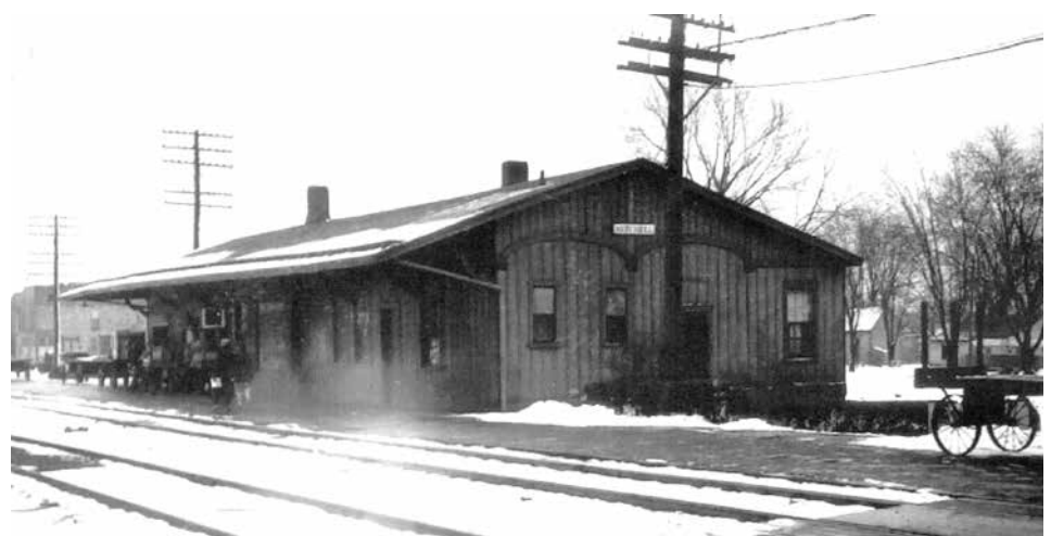
Taken in the 1940s, this is a view of the west end and front of the original O&M/B&O passenger depot in Mitchell, Indiana, looking east. This end of the depot, built around 1857, contained the waiting rooms and the ticket agent's office/operator's bay. A random snowflake may account for the blur in the image. (Robert Clark collection, BORHS)
