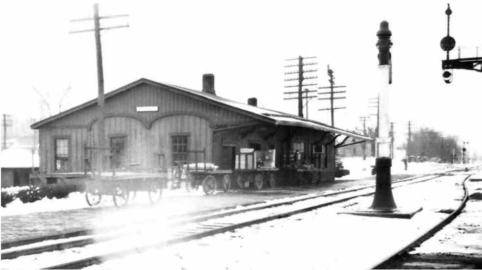
This view of the east end and front of the Mitchell O&M/B&O passenger depot apparently was taken the same day as the one on page 5, with the same camera. This end of the depot contained the freight/express room, and a baggage room--originally a lunchroom. There was an additional penstock at the west end of the platform.
