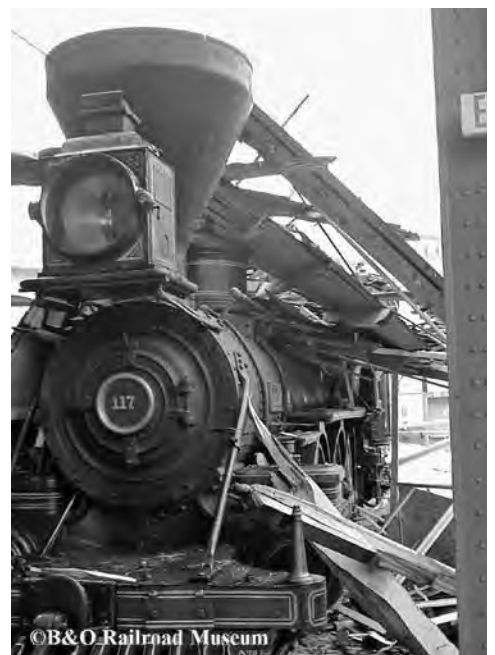
One more look at the locomotive the day after the roof collapsed, before the debris was cleared away.
