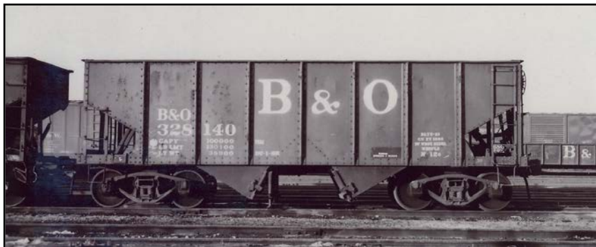
328140 Willard, OH left side, January 30, 1965 Julian W. Barnard Coll., B&ORRHS Built 5/23, Pressed Steel Car. Note brake reservoir bracket and location of slope sheet braces. Ajax power hand brake visible on right side. I believe the white dot means the car is suitable for carrying powdered coal.
