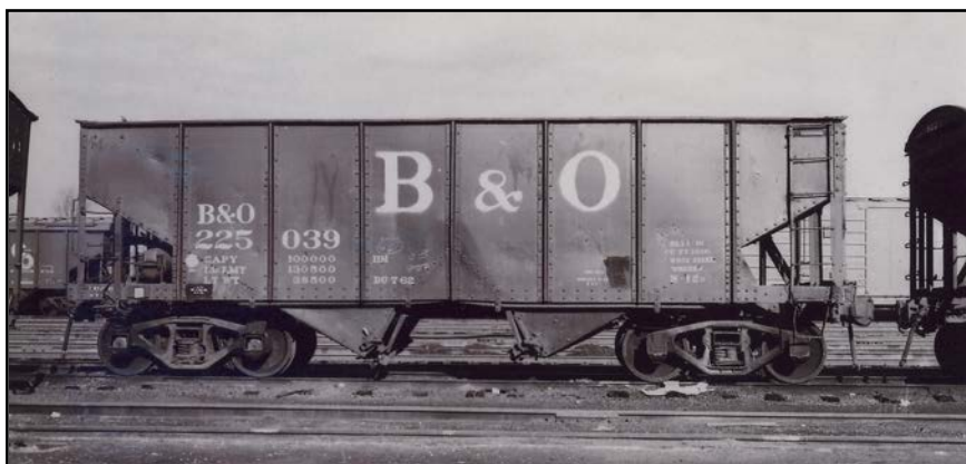
225039, Willard, OH right side, December 14, 1964 Julian W. Barnard Coll., B&ORRHs. Note outside air line and damaged left sill step. Wine door locks
