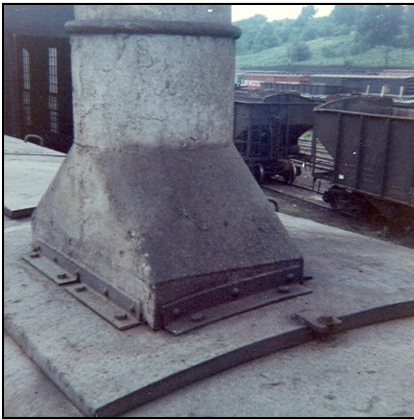
Detail view of stack; notice angle irons at base.
