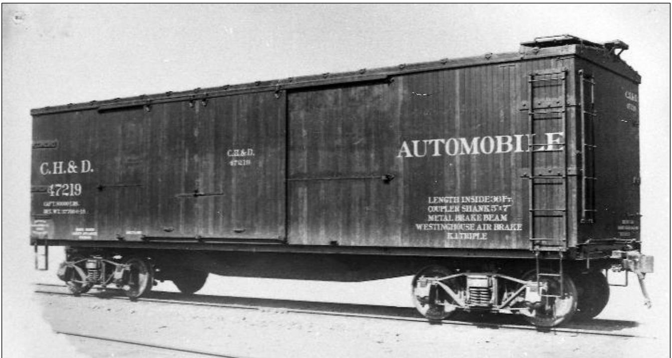
The CH&D also installed 500 automobile boxcars from American Car & Foundry in 1915. Except for the door openings, the automobile and boxcars had the same dimensions. AC&F photo
