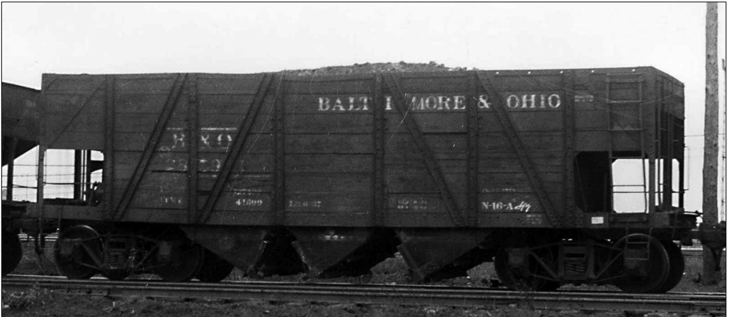
The N-16 and N-16a cars were distinctive, as you see above. They were wood construction with steel underframes and truss members following a Seley design. The B&O was rebuilding these cars in the mid-1920s with steel hoppers, steel ends and open sides under the slope sheets at the end sills.
