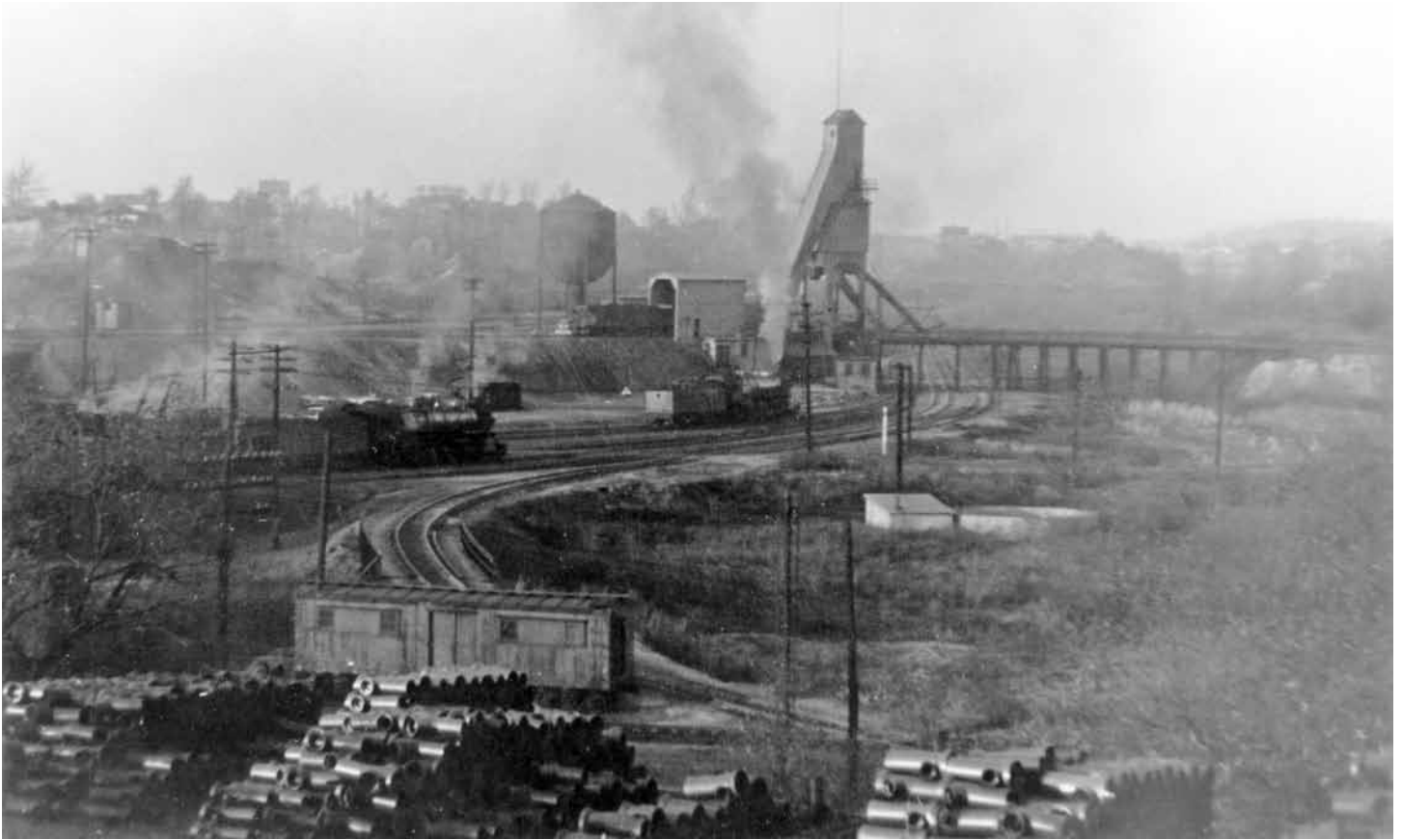
We are looking northeast toward the west end of Hill yard and the coaling tower at Akron Junction, Ohio, sometime in the early '50s. Though locomotives are smoking up our view, we can see the water tank and coaling tower with the Loop line trestle crossing over the Pittsburgh, Cleveland & Toledo Railroad and the wye track, which curves off to the right under us. The Valley main would be just in front of us, hidden below that boxcar that looks like a derelict B&O car. (Edwin C. Kirstatter collection)
