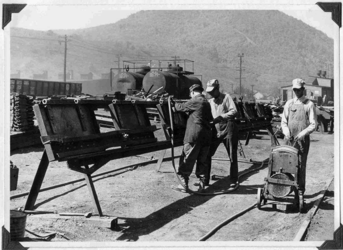
Hopper Doors fabricated in advance of requirements on special convenient racks.
