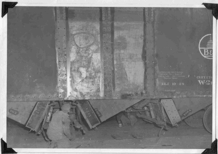
Car then moves to Spot "D" inside the barn, where the work of reaming and driving body above underframe is accomplished.
