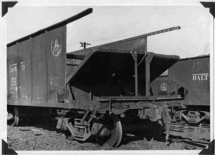
Spot "A" - Here cars are given a very thorough inspection, defective parts are removed, trucks are removed and sent to a special truck spot for overhaul. Cars are placed on trestles and parts requiring renewal are replaced.
