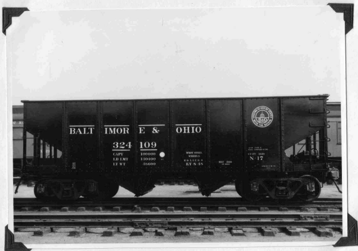
Spot "F" - After the second coat of paint is applied, the car is stencilled, and car is again serviceable and ready to go back to the transportation department for many more months of service.
