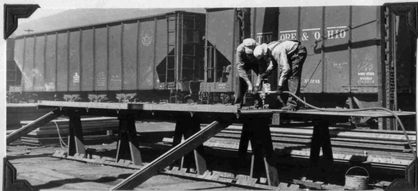
Rivet holes are reamed, and sheets formed in a single unit.
