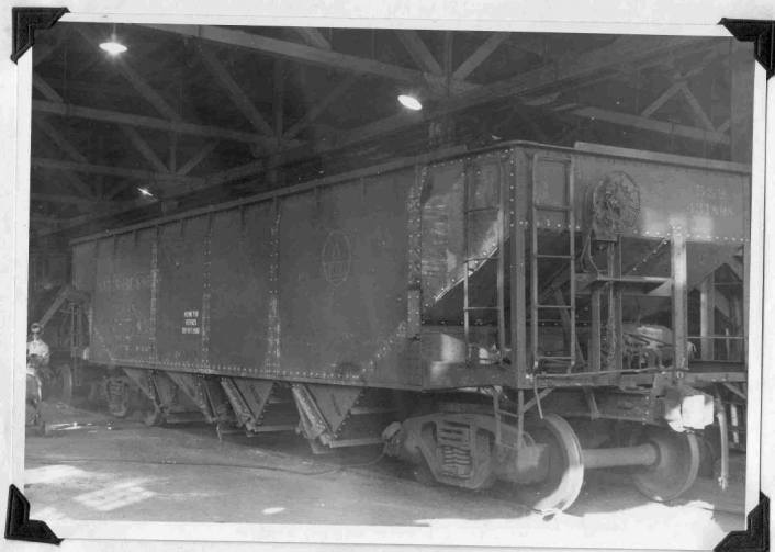
Spot "F" - Safety appliances are installed, doors are hung, and car is ready for application of AB equipment.
