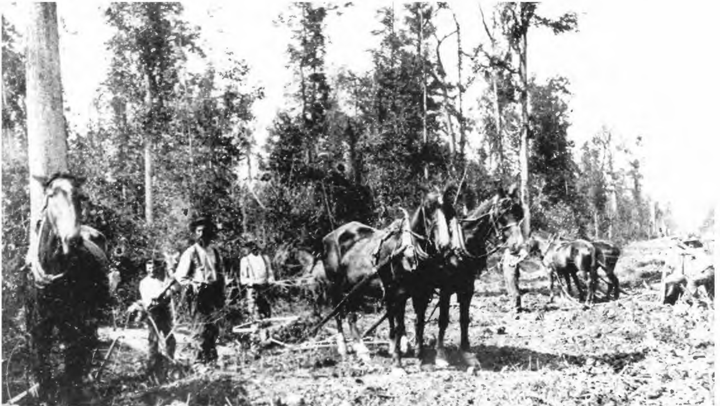
Peat bogs were found on much of the route of the Chicago Division, such as this area near Deshler, Ohio, being cleared for the right of way in 1873. 396 trestles were required to cross the "puddles" which, if laid end to end, would have extended nine miles. (Photograph courtesy of Patrick Henry School District Public Libraries, Deshler, Ohio)
