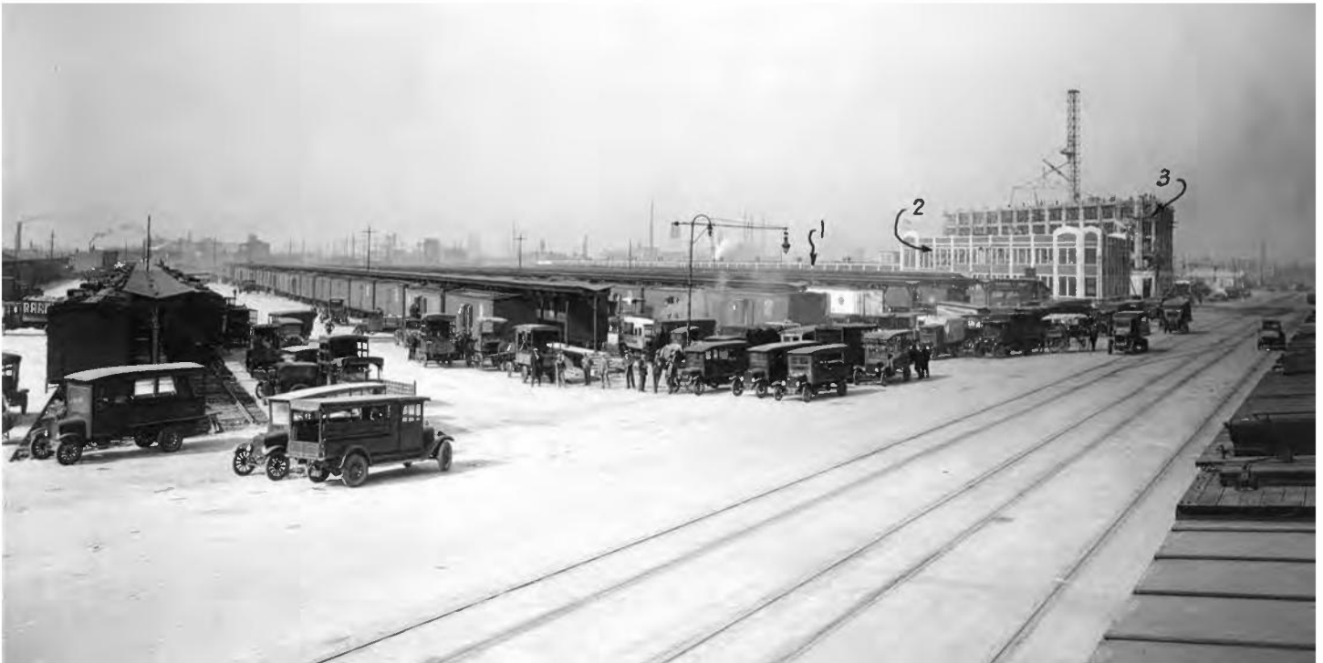
Taken from the top of a box car looking north along Delaware Avenue, the Auction Sales Shed (1) and the Auction Sales Building (2) are in full operation while the Cold Storage Warehouse (3) is still under construction. (B&ORHS Archives)
