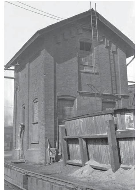
The massive frame coal elevator and the brick sand house at the Washington engine terminal are shown in these ICC Valuation photos from about 1918. The coal facility was set up to serve two locomotives on each side. The sand house had an elevated tank for dry sand at its northwest corner.
