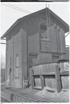
The massive frame coal elevator and the brick sand house at the Washington engine terminal are shown in these ICC Valuation photos from about 1918. The coal facility was set up to serve two locomotives on each side. The sand house had an elevated tank for dry sand at its northwest corner.
