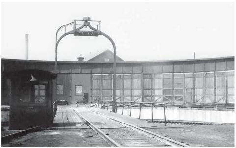
The B&O roundhouse and turntable at the Washington engine terminal, shown here in about 1930, probably were built at the same time as the Shops. This 100-foot turntable replaced the original 70-foot turntable around 1918. (Robert Clark collection, B&ORHS)
