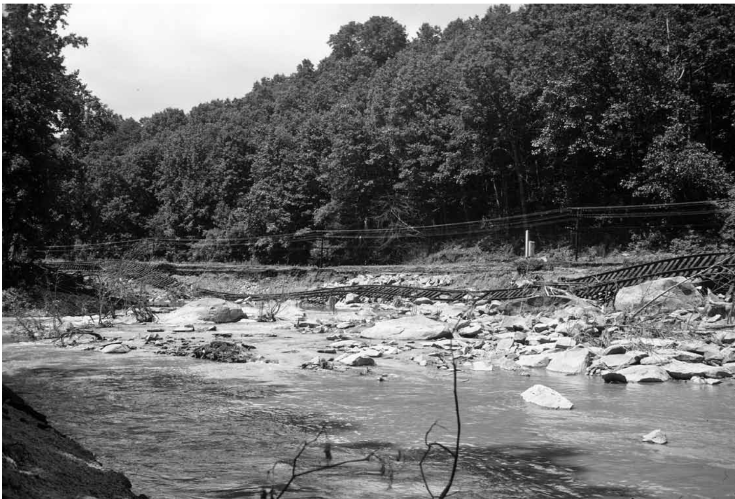
Twisting through its channel, the Patapsco River undercut Old Main Line roadbed at every turn. As in so many other places, this segment of track east of Sykesville was left dangling and twisting when the flood receded. East of Marriottsville, a 300-foot segment of roadbed 50 feet wide was lost. East of that a section 25 feet deep and 90 feet across disappeared. (John King photograph)
