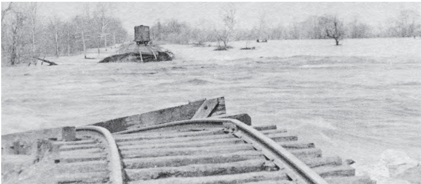
The scene of the washout at Blue Hole Pond in southwest Indiana on March 27, 1913. Four men died when a locomotive went through the 230-foot-long trestle, and the 150 workmen in the cars remaining on the tracks were stranded when the White River Bridge farther west was also washed out. (All photographs, Chas. E. Smith collection)
