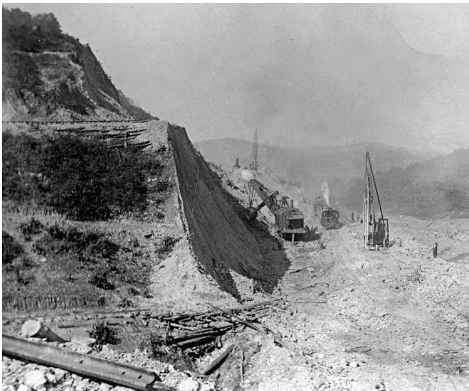
The magnitude of the construction of the Magnolia Cutoff required a huge amount of manpower and equipment to make it possible. A total of 22 steam or air shovels were used on the project with 19 Marion, two Marion Osgood and one Bucyrus shovel being employed. On most of the sidehill work, steam drills were used while air lines were installed for the tunnel work and the work at Doe Gully Cut. A total of 66 air drills and 50 steam drills were needed. The photo shows an air-operated Marion shovel employed for use in the tunnels. (Photo previously appeared in East End: B&O's "Neck of the Bottle" )
