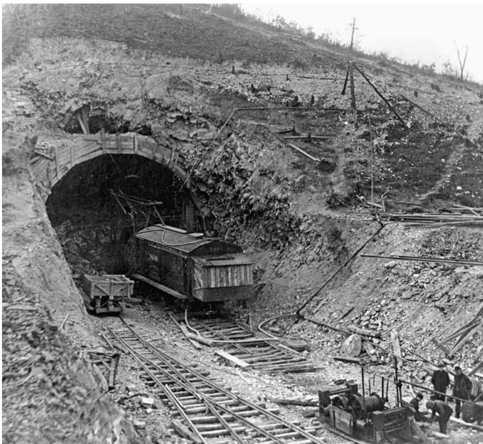
The magnitude of the construction of the Magnolia Cutoff required a huge amount of manpower and equipment to make it possible. A total of 22 steam or air shovels were used on the project with 19 Marion, two Marion Osgood and one Bucyrus shovel being employed. On most of the sidehill work, steam drills were used while air lines were installed for the tunnel work and the work at Doe Gully Cut. A total of 66 air drills and 50 steam drills were needed. The photo shows an air-operated Marion shovel employed for use in the tunnels. (Photo previously appeared in East End: B&O's "Neck of the Bottle" )
