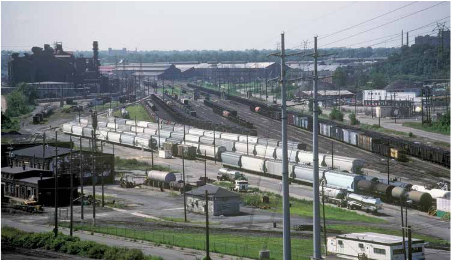
The west end of Clark Avenue yard looking south. In the center foreground is the BIDS (Bulk Intermodal Distribution Services) terminal area filled with covered hoppers and tank cars with loads waiting to be transloaded to trucks. The small gray structure at bottom center is the old west end yard office. (Ron Spiga photograph, September 1990)
