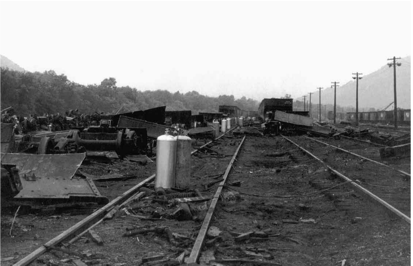
Things get a bit cluttered along a railroad Repair in Place, or “rip” track, as this one at Brunswick demonstrated. Note the number of gas canisters, probably for welding or burning jobs, and the pieces of scrap metal all over. The job of the day appears to involve hopper cars. (Brunswick Heritage Museum collection)
