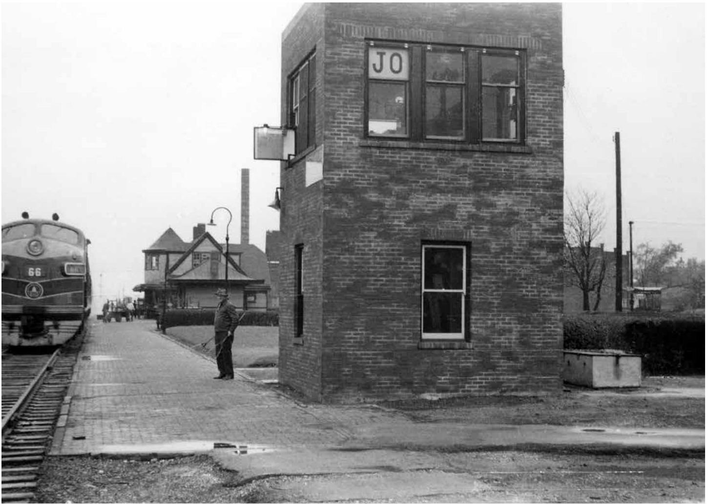
Compare this photograph with the one on page 3. The watchman's shanty at the B&O/PRR crossing is gone, replaced by JO Tower, whose operator waits to hand up orders to a westbound passenger train around 1950. The tower, built in 1949, remained in service until 1991. (B&ORHS, Robert Clark Collection)
