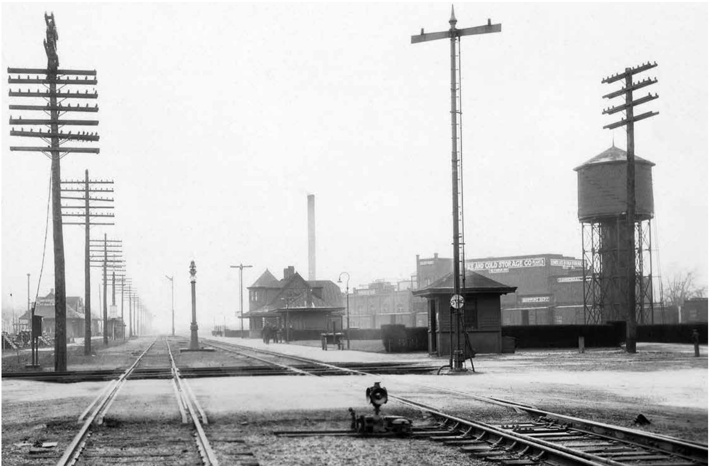
A watchman stationed in the shanty at the right-center of the photograph operated the tilting target signal to control train movements at the B&O/PRR crossing in Seymour, Indiana. He also controlled the movement of motor vehicles at the grade crossing. By the time this photograph was taken, around 1930, the roundhouse and coal dock had been removed. The Ebner Ice & Cold Storage Company is visible behind the shanty. The Milwaukee (SIRR) depots are on the far left.
