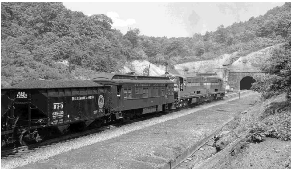
B&O used 930 to evaluate the Fairbanks-Morse H-24-66 Trainmaster demonstrator units in 1953, and chose not to buy any.
