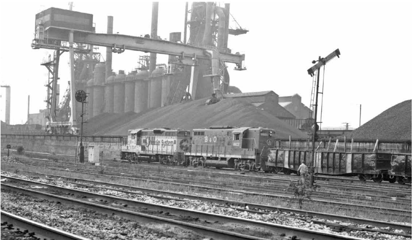
An eastbound B&O train passes one of Republic Steel's furnaces in Youngstown, Ohio, in the 1960s. Note that one of the diesels is a former passenger GP-9, distinguished by the "torpedo" air tank atop the body. In the foreground is A-Bros Crossover, of which more later. A color position light signal and semaphore help control traffic here. (Don Riel collection)
