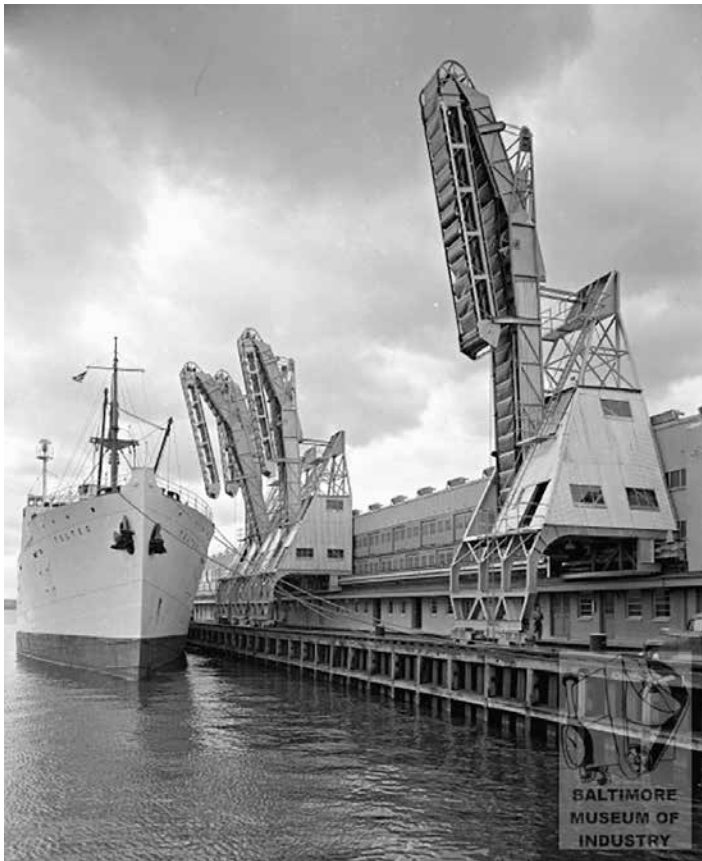
[below and right] These two photographs show the conveyors used to move the bananas for loading into railcars.
