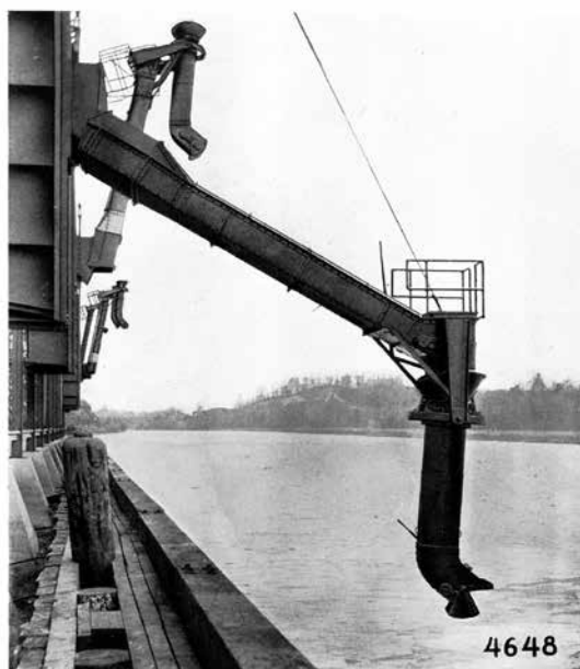
View of Adjustable Loading Chute in Operating Position
