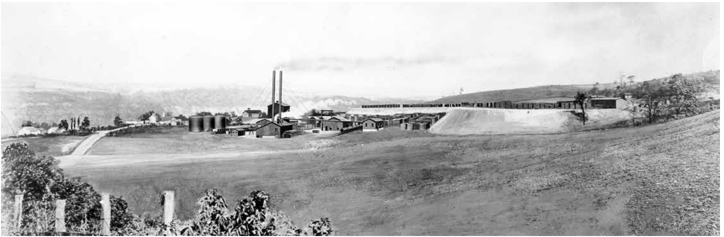
This appears to be a postcard view of the Adelaide, Pennsylvania, tie treatment plant, probably from the early 1900s. To the right side of the image, finished ties are being stored on a large area of fill.
