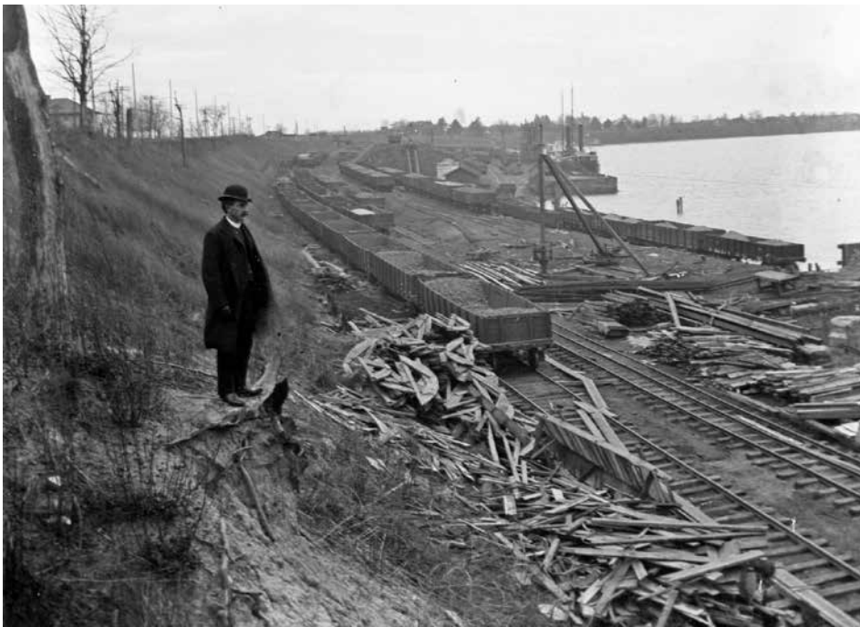
The Rossford Dock site looking south about 1900. The grain elevator has burned, and it appears they are extending the track north to supply construction material for the building of the new NYC bridge over the Maumee River. The three tracks left served the B grain elevator, and its replacements. They are in similar arrangement even today. In the distance, more tracks serve the ore and coal dock, with a large pile of material stored on the ground between the two. (Toledo Lucas County Public Library)
