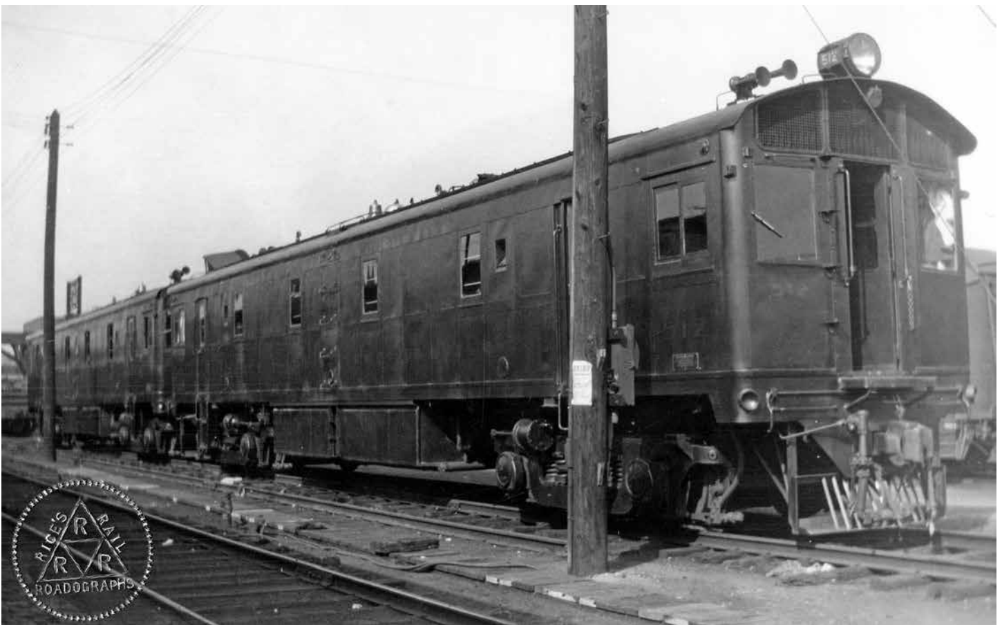
EMC Demonstrators, EMC 511-512, DP-1, diesel, Electro-Motive Corporation, circa 1935, possibly Camden Station.
