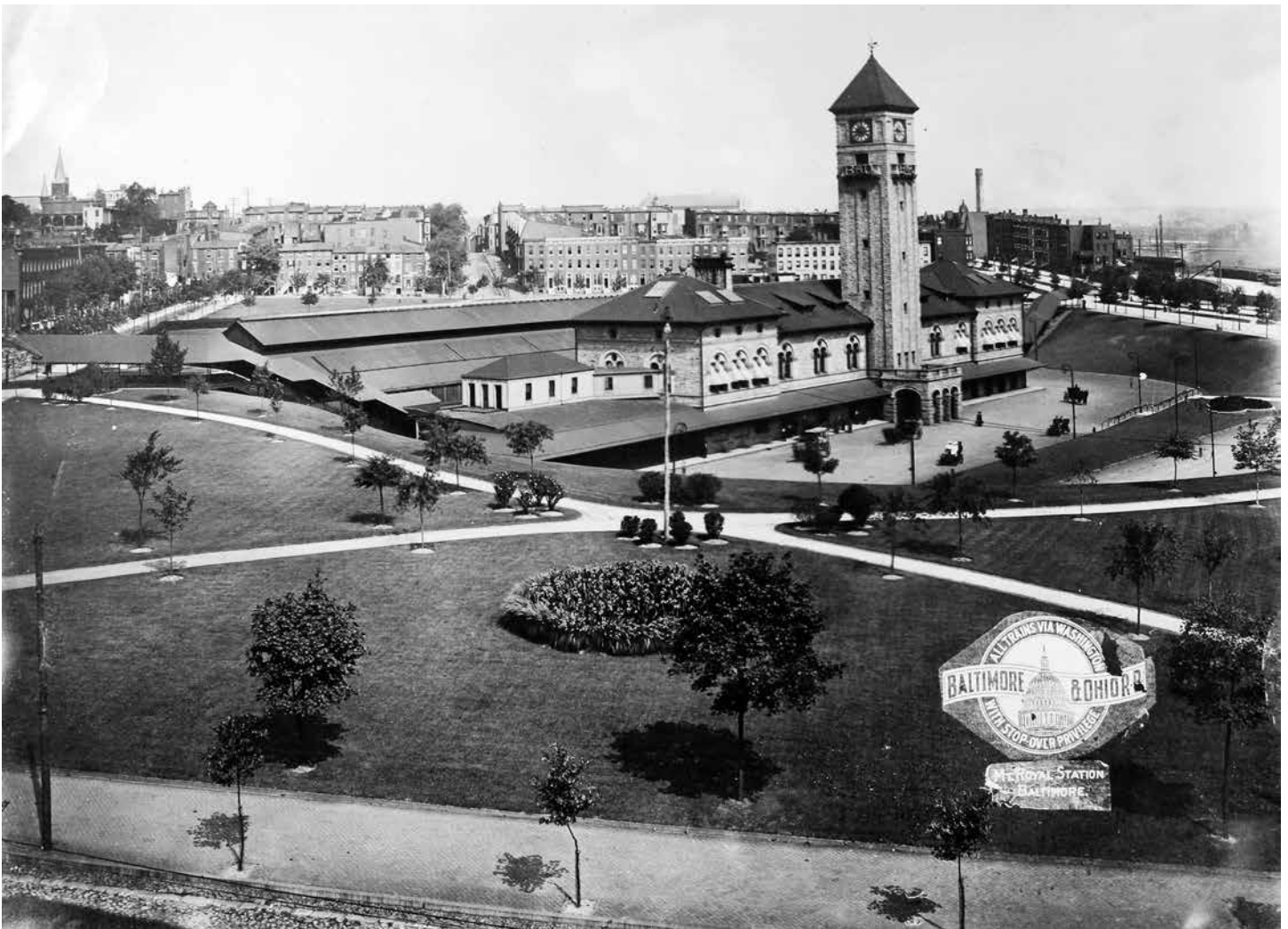
Exterior view of Mount Royal Station with B&O seal. (ICC, Bureau of Valuation, Engineering Field Notes, located at the National Archives at College Park)
