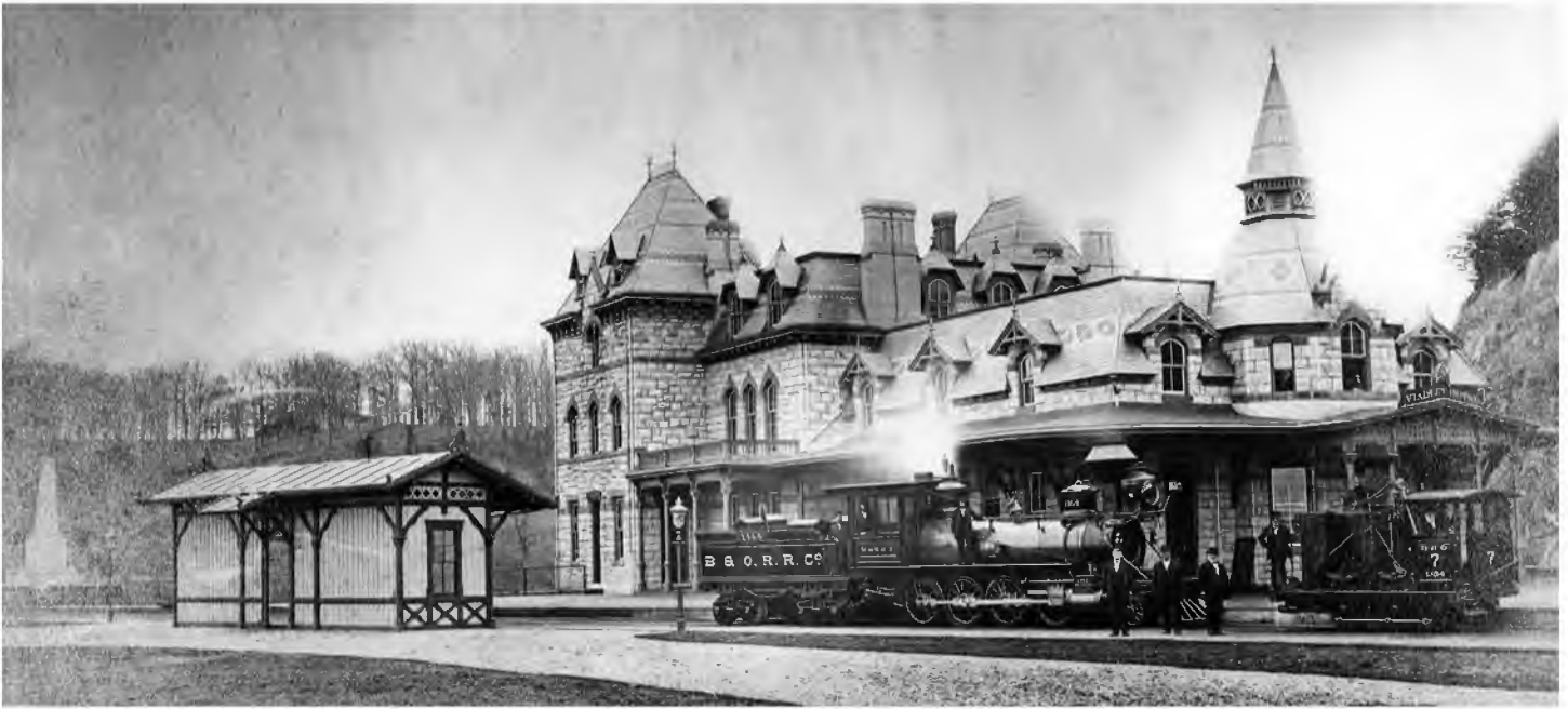
Opened in 1873, the E.-Francis-Baldwin-designed Viaduct Hotel in Relay, Maryland is six miles west of Baltimore. This staged photograph includes the then-oldest surviving B&O engine, a so-called grasshopper-type sporting an 1834 date, and its newest engine, a much larger 2-8-0. The original mainline ran behind the hotel. The Washington Branch extended to Washington in front of the building. The station was on the east (right side) of the building.
