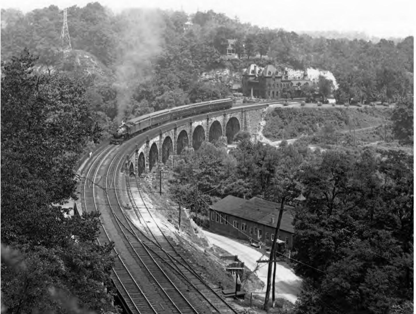
The Viaduct Hotel is on the bank of the Patapsco River where the Washington Branch leaves the original mainline and crosses the Thomas Viaduct.
