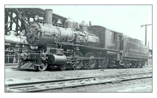
The subject of my model 1373 is shown here at Parkersburg, WV on August 11, 1940. It is one of the B-8 class built by Baldwin Locomotive Works in 1893, now modernized with electric headlight, steel cab and larger tender. According to *Steam Locomotives of the Baltimore & Ohio, An All-Time Roster* by William D. Edson, 1373 was scrapped in August of 1947. Edwin Kirstatter's Collection.
