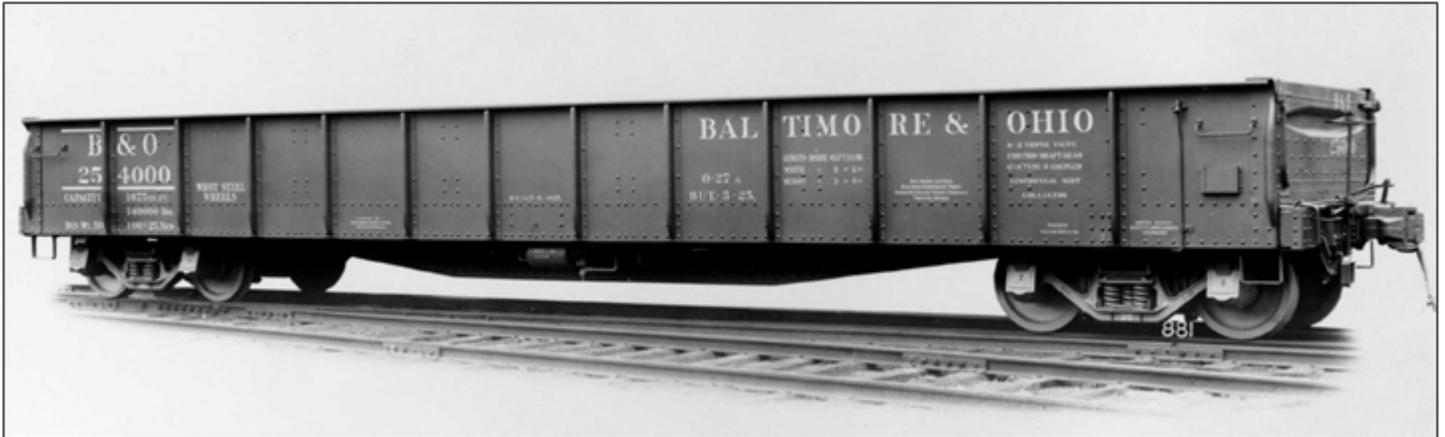
O-27a 254000 in a Standard Steel Car Company builder image from May 1925.
