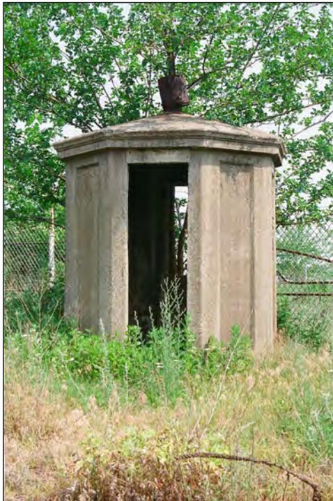
Booth on north side of tracks and west side of Newkirk St., straight-on view of door side. Note intricate cornice detail and collapsed sheet metal smoke jack. 6-01-11
