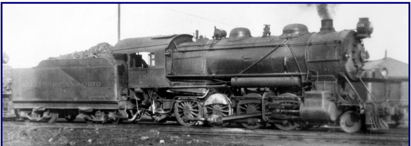
B&O 2501, Class E-27, built by ALCo (Schenectady) in 1905-06. Converted to B&O 605, Class L-2 in April 1925. Renumbered to B&O 1605 in 1954, retired in 1955. Baltimore MD, date unknown (Max Miller photo).
