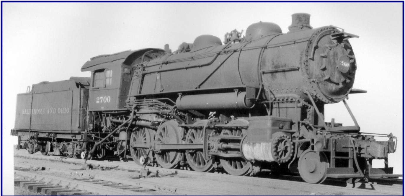
B&O 2700, Class E-27, built by ALCo (Richmond) in 1905-06. Converted to B&O 710, Class L-2C at Mt. Clare, May, 1931. Renumbered to B&O 1623 in 1954, B&O 839 in 1956, retired in 1957.
