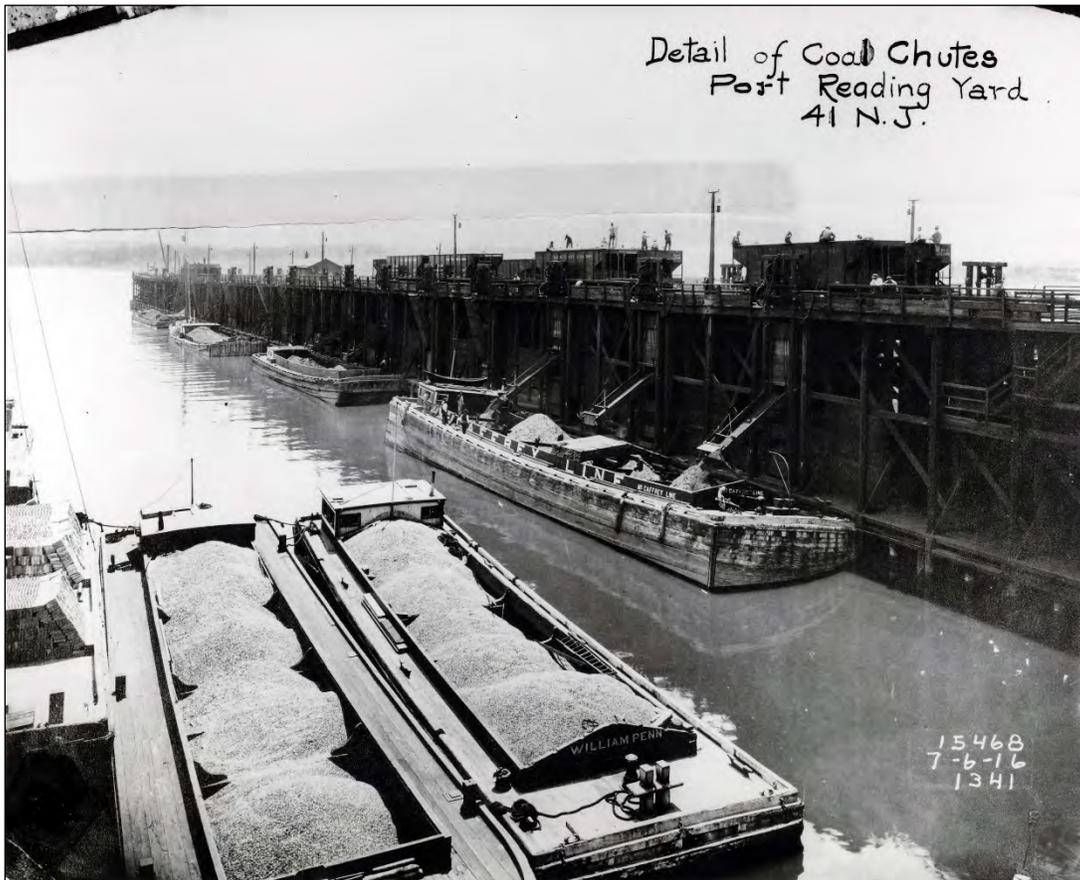
N-13s unload at Port Reading coal trestle on Arthur Kill, 7/6/16, photographer unknown. Note the abundance of manpower in use to facilitate unloading.
