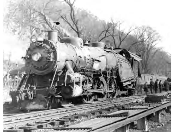
Engine 5218, a P-5 built by Baldwin in July 1919, was much the worse for wear after rolling onto its left side at 48 mph and sliding the equivalent of three football fields. But it was rebuilt as a P-5a in December of 1928 and remained in service until October of 1956.
